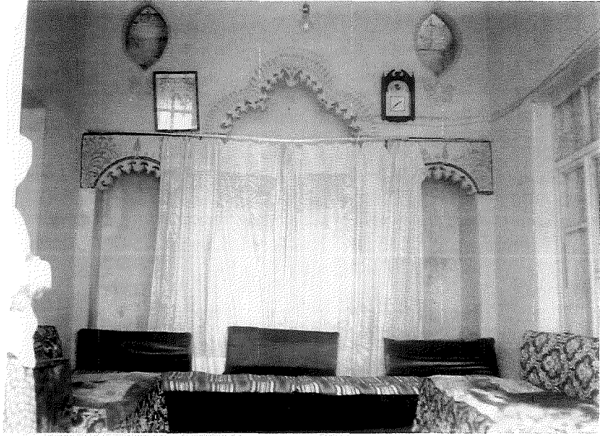
Figure 25 Summer "eyvan" in Ibrahim Paşa House. The two niches at the rear wall are connected to the ventilation channels leading up to the roof.
