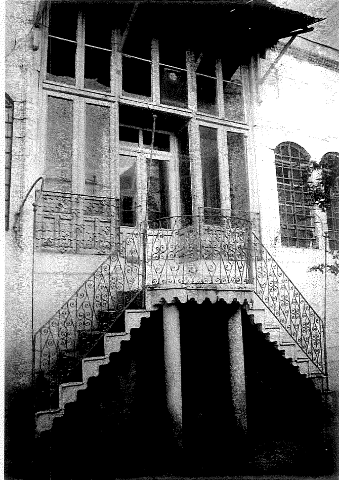
Figure 34 Curvilinear iron balustrades of the staircase in Kaplama House.
