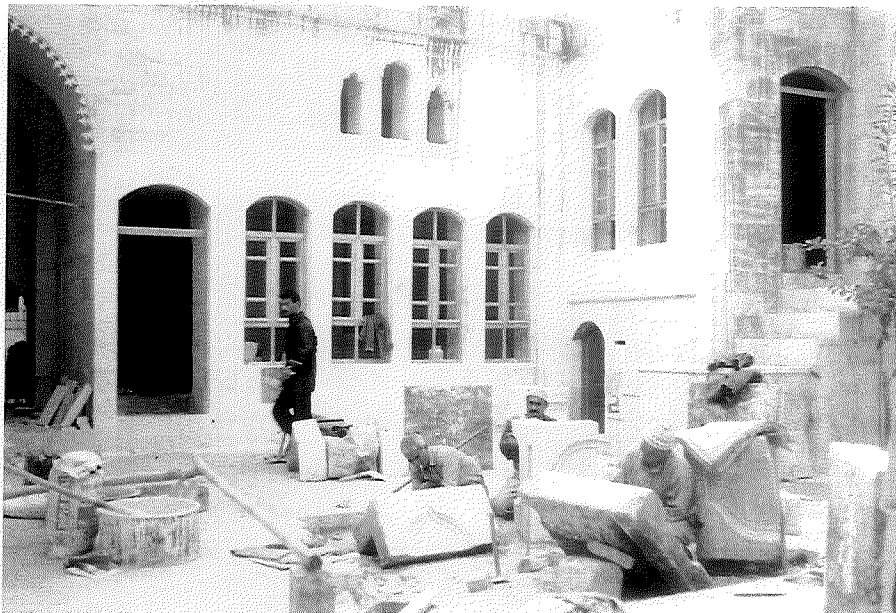
Figure 31 Stone masons working in restoration of a traditional house.
