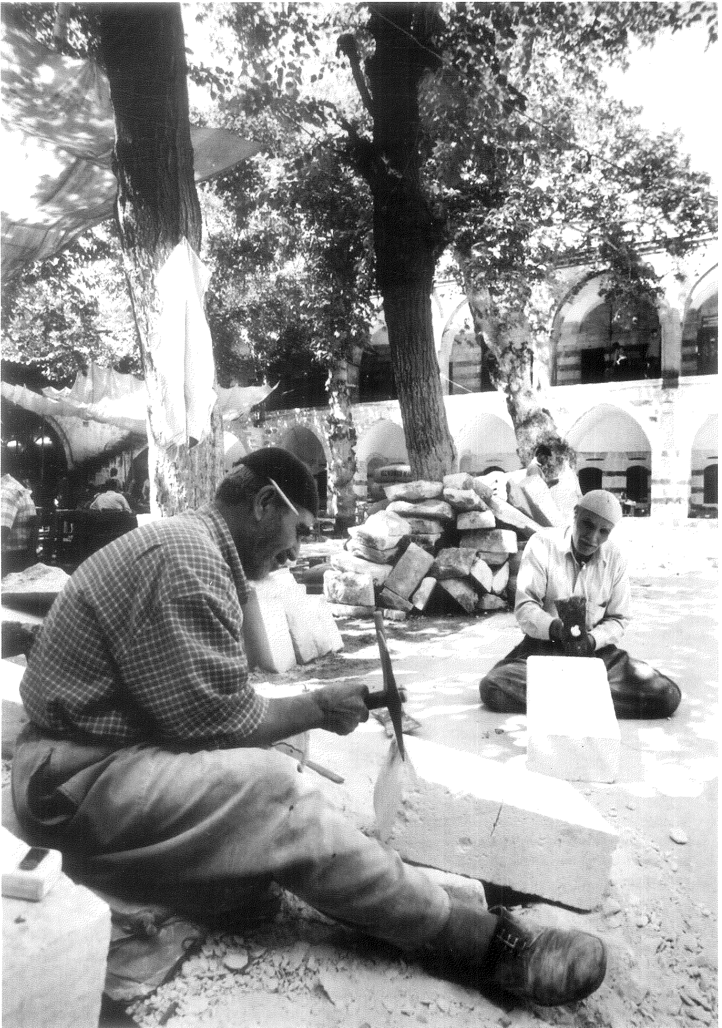
337) Stone dresser in Gümrük Inn renovation. (Photograph by: A.Cihat Kürkçüoğlu / 2001).
